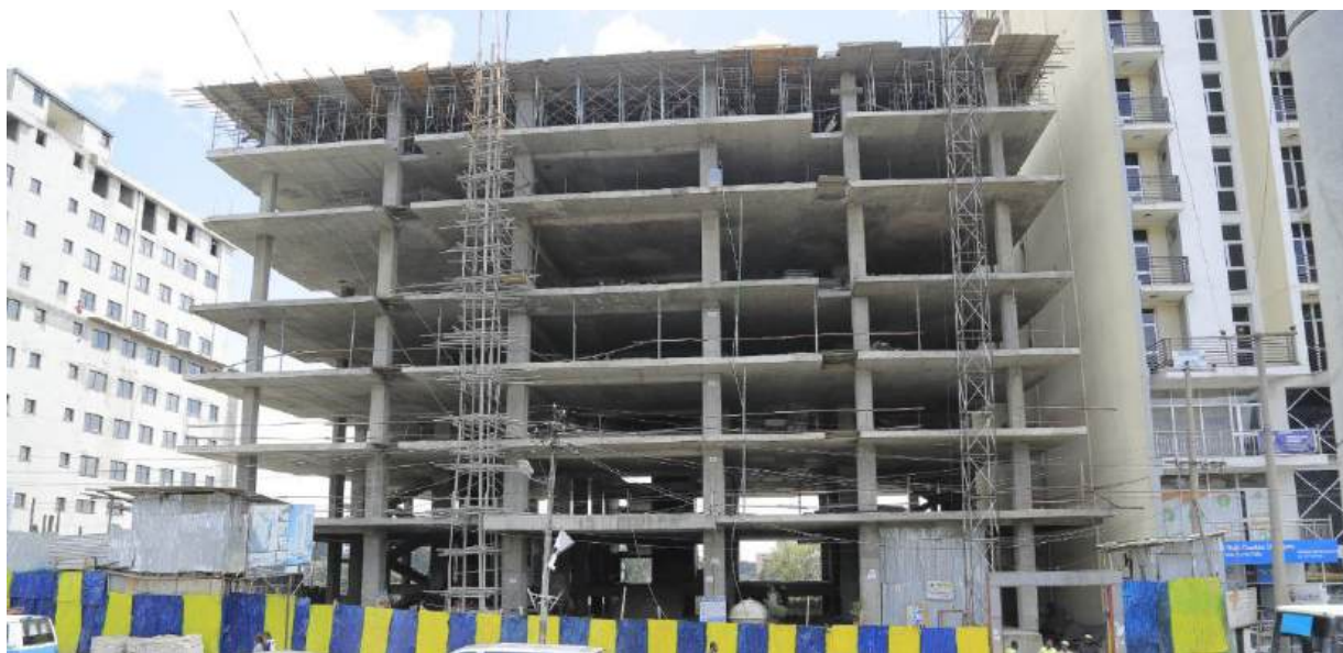
Partial View of the Construction of the Head Quarter Building
